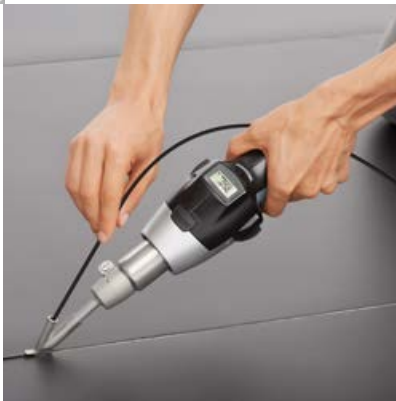
▼ Welding linoleum floor HG 2620 E
