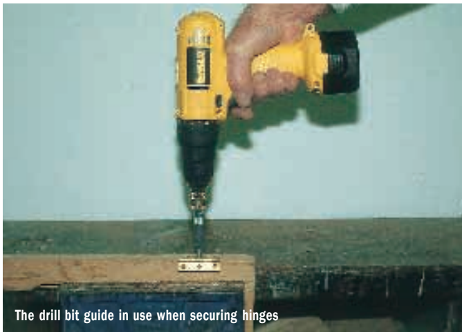
Boring with a twist bit
